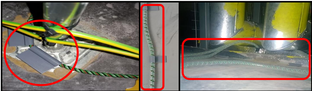
Figure 14: Use Hold down clip to separate the sensing cable & Use PVC spiral sleeve to wrap round the affected length of the sensing cable
